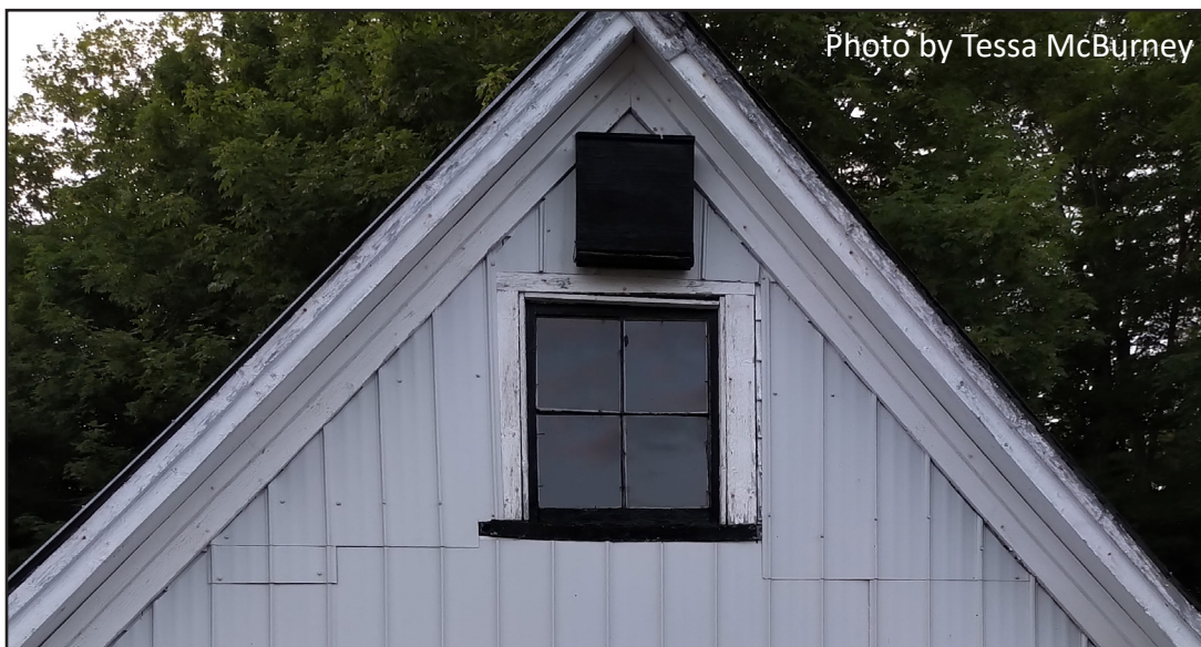
Figure 60. Bat house on a shed.
